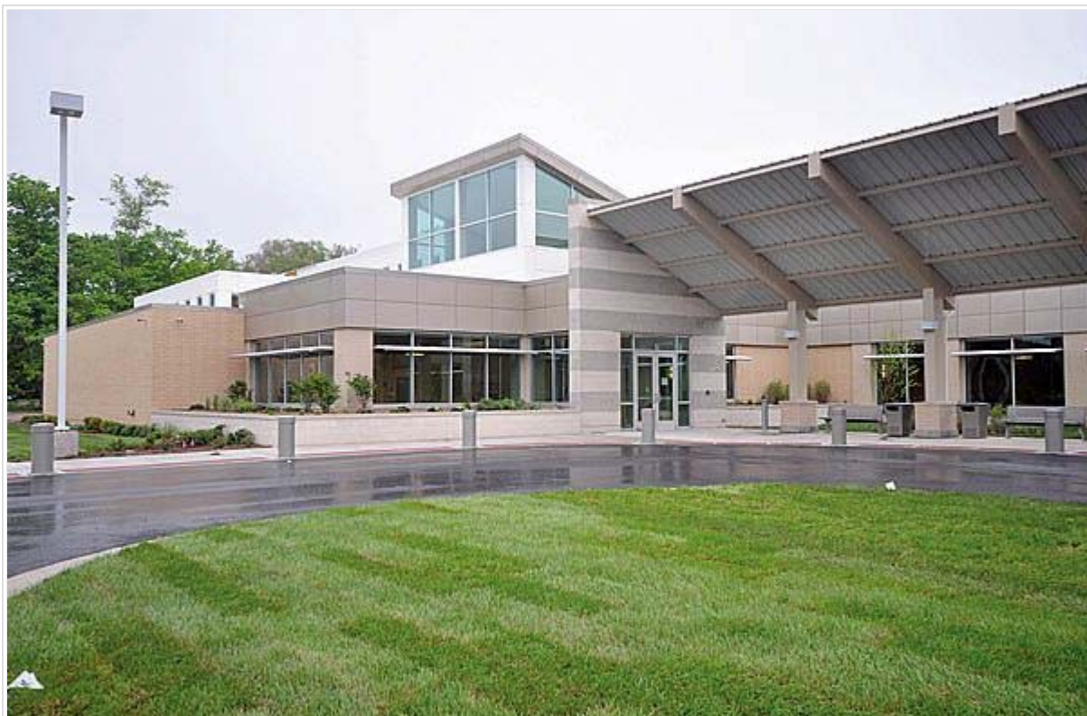
This is the main entrance to the new clinic. John Madill / H-P staff
